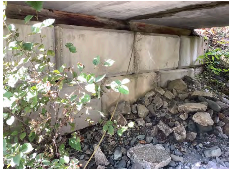
Right Bank Abutment when facing downstream
