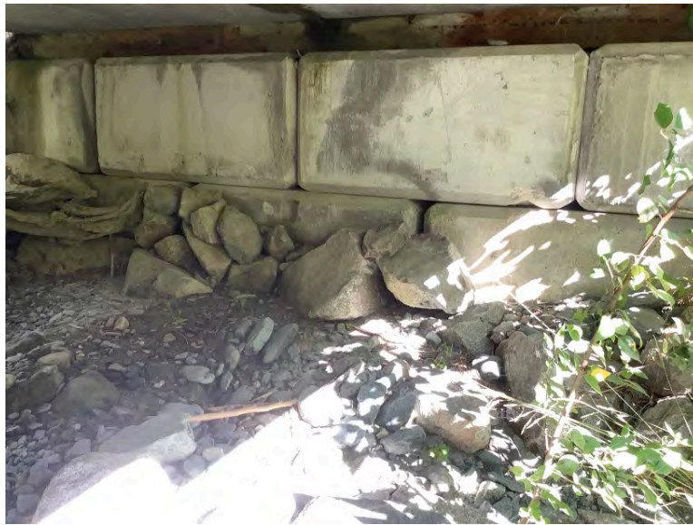
Left Bank Abutment when facing downstream
